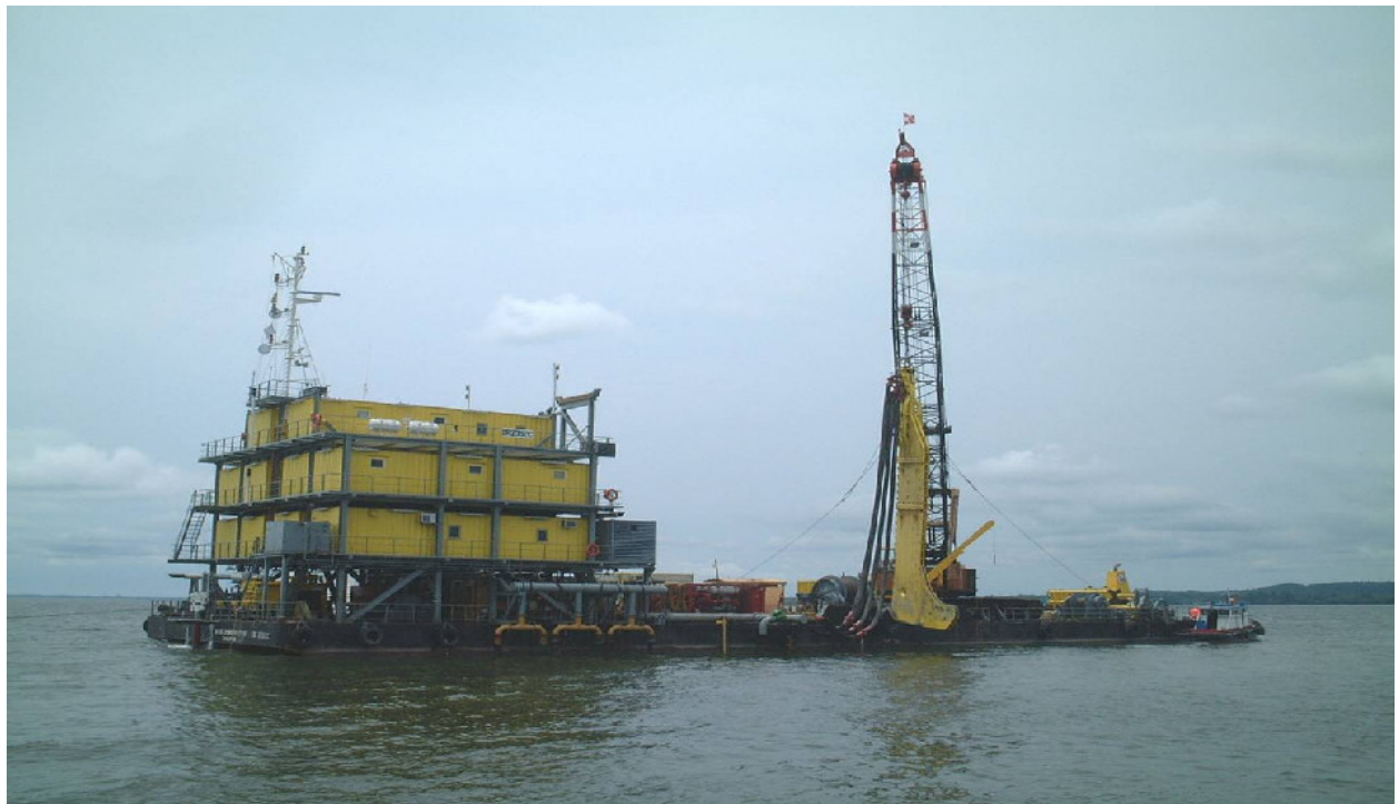
Cable laying barge with injector tool 裝有注射工具的光纜鋪設躉船
