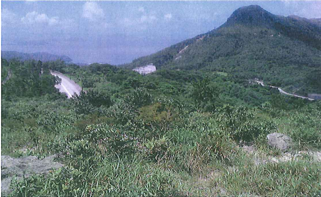
Picture 2: General view of surrounding area to the northwest of the Integrated Mobile Phone Base Station
