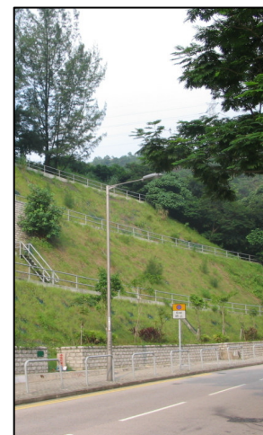
Examples of green slope with soil nail installation and existing tree retained after landscape treatment
