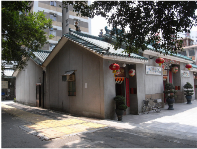
Figure C1d – Tin Hau Temple, Tai Po Kau Hui (Grade III)
