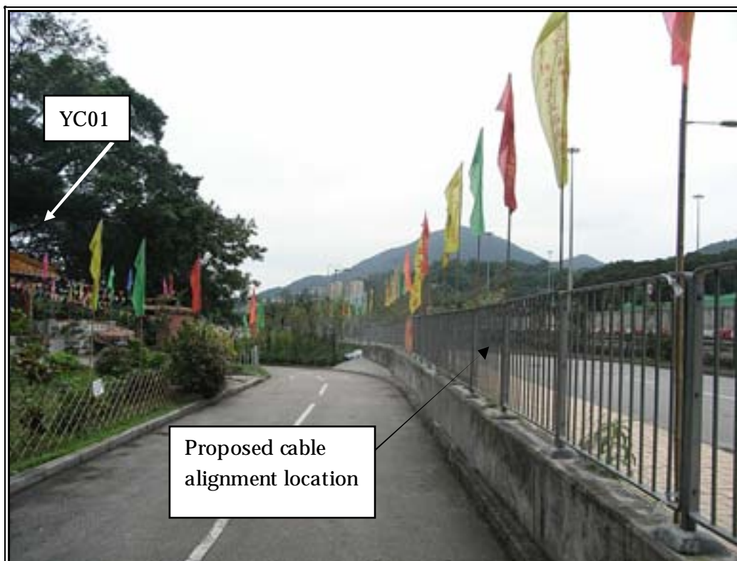
Box 4.1 Photo showing YC01 Location and the Proposed Cable Alignment.
