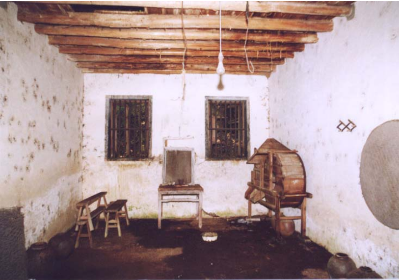
Photo 3 Main Building Ground Floor (Main bay) 相片 3 主樓地下(明間)
