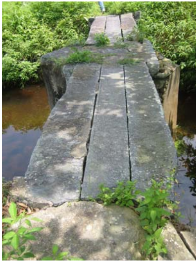
LMH-01 Old Bridge, Lin Ma Hang, Sha Tau Kok, N.T.
