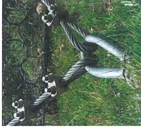
Views of the anchors
