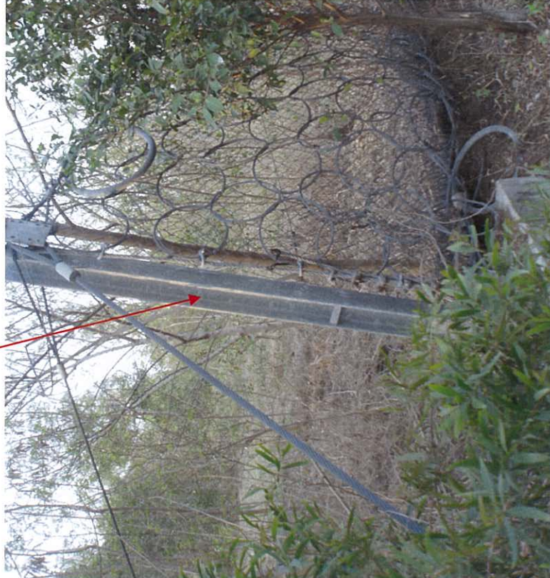
Close-up View of Flexible Mesh and Supporting Post
