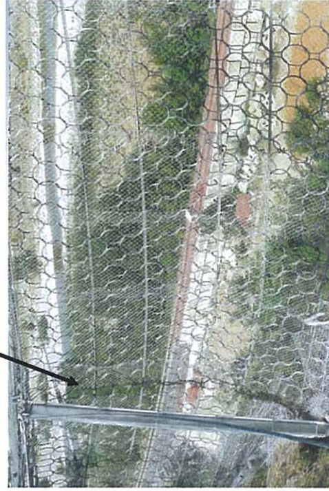
View of proprietary flexible barrier after installation
