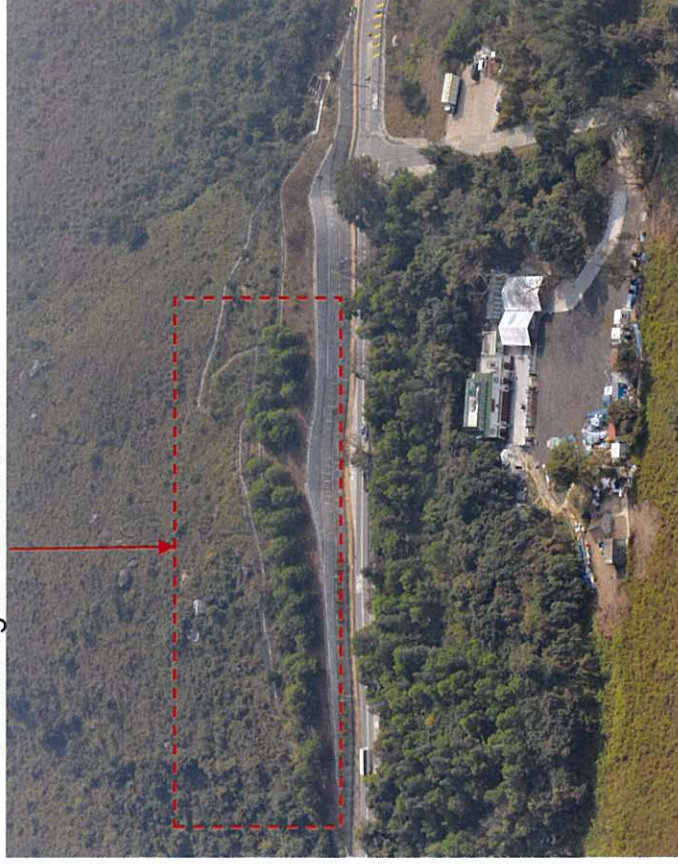
Plate 5a – Aerial View Showing Pit-planting in front of the flexible barrier for screening (Example: Tung Chung Road)
