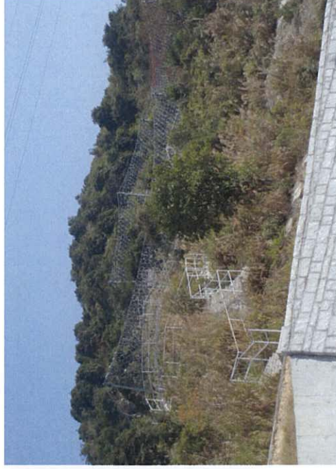
View of Flexible Barriers Close to Roadside of Tung Chung Road
