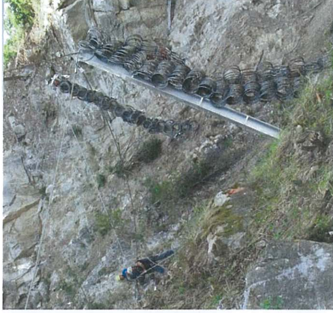
Example of installation process of the proprietary flexible barrier
