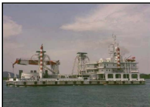
Typical Cable Installation Barge using Injector Burial Tool
