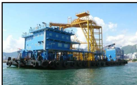
Typical Cable Installation Barge using Sledge Tool
