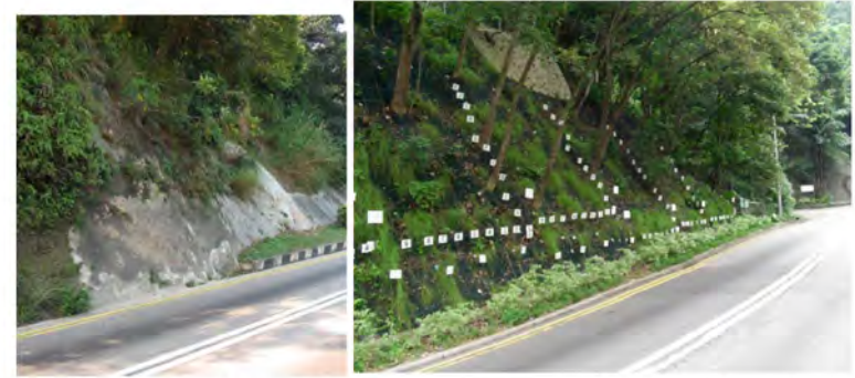
Before slope upgrading works
