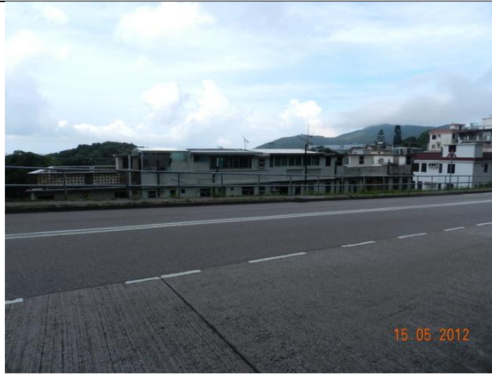
VP11 – Located at the slope toe of the existing hillside woodland; only the top floor and the roof of the village houses in Sheung Yueng area are above Clear Water Bay Road
