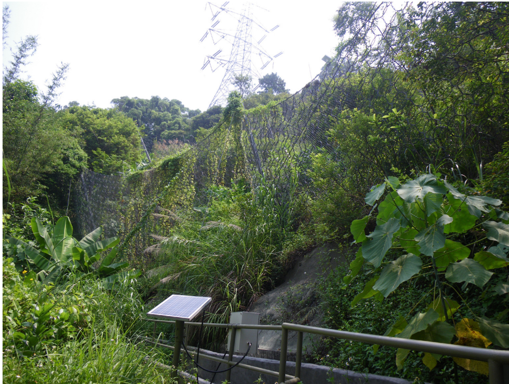
View of Flexible Barriers and access with painted handrails
