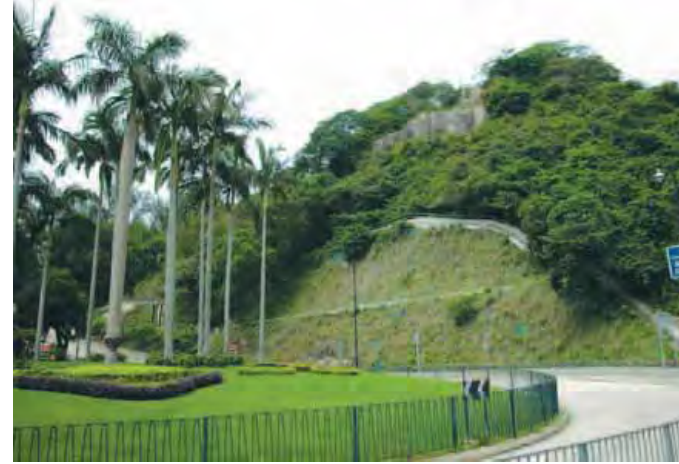
Slope installed with Soil Nails (at completion of upgrading works)
