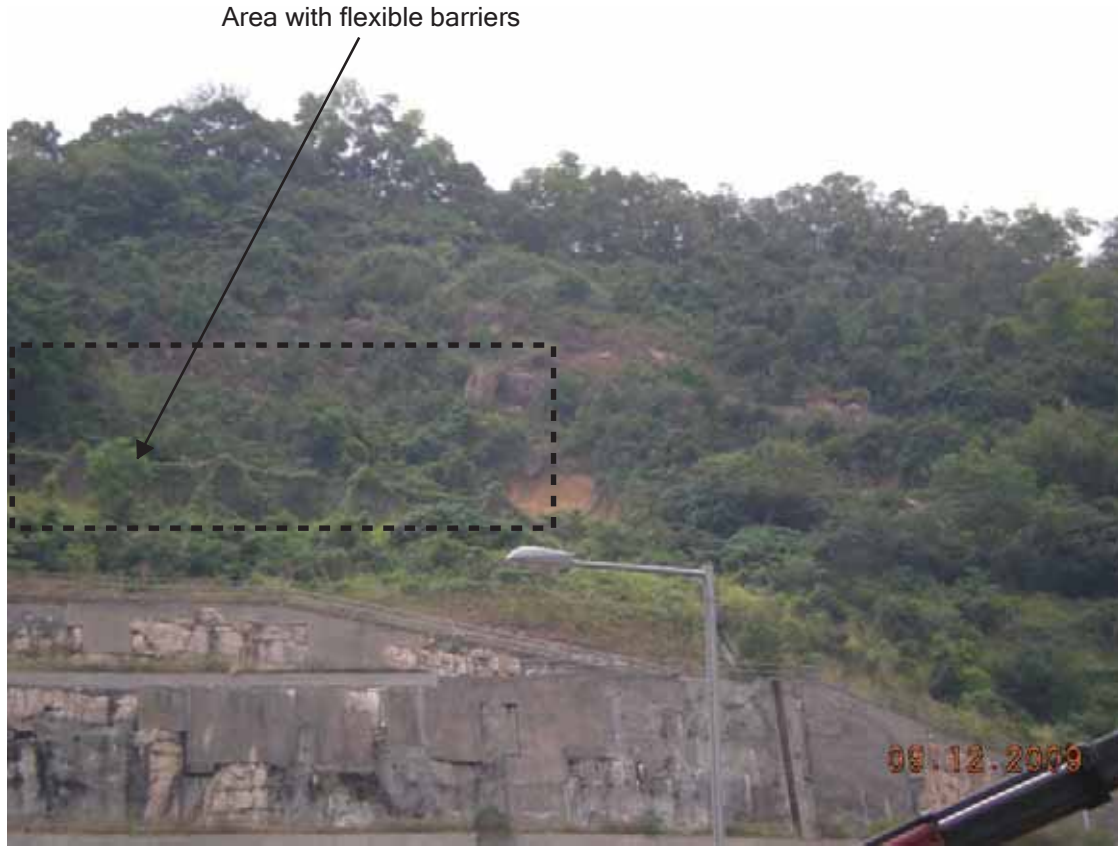
General View of the flexible barrier
