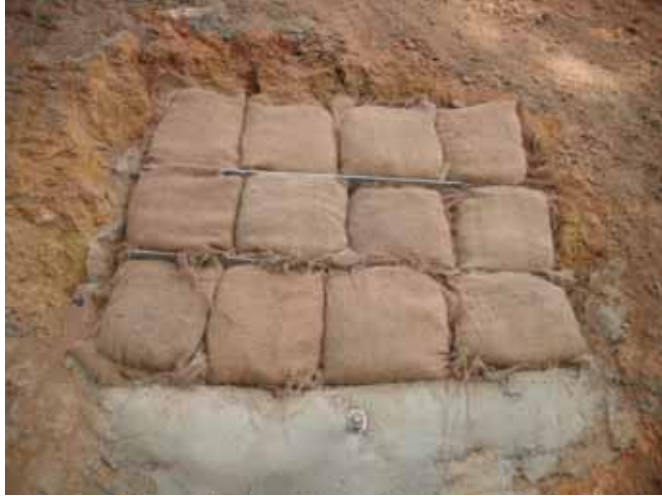
Example of Completion of Soil Nail (Head)
