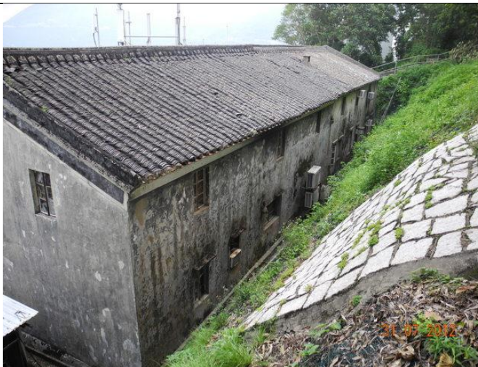
VP11 – Located to the southeast of the Works Area and the topography of the existing man-made slope is higher than the adjacent village houses
