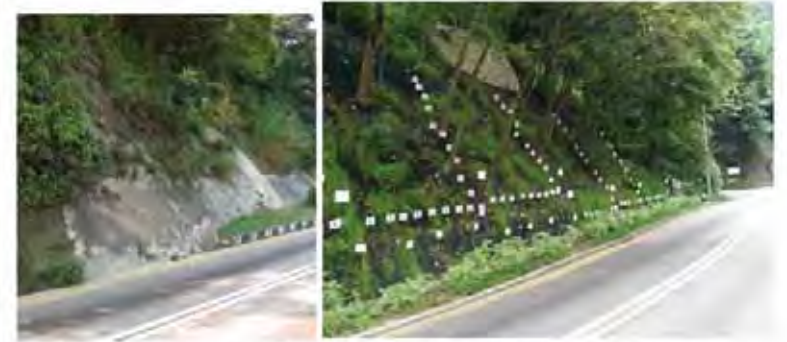
Before slope upgrading works
