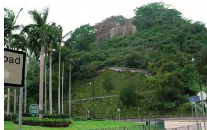
2 years after completion of upgrading works
