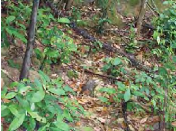
Close up view of the works area
