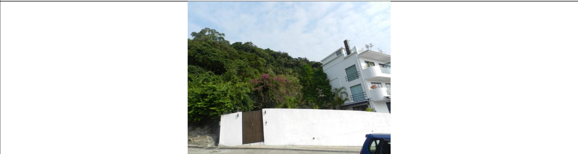
VP4 – Overall view of the western part of the proposed slope work within the woodland area. The maximum height of the slope (Slope Feature No.: 12SW-A/CR 45) adjacent to the village house is 16m and the presence of the existing vegetation also block the view of the slope works within the woodland
