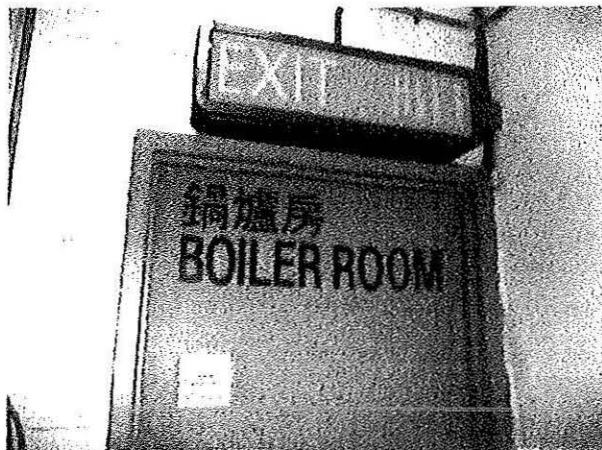
Photo 16. The Entrance of the Boiler Room.
