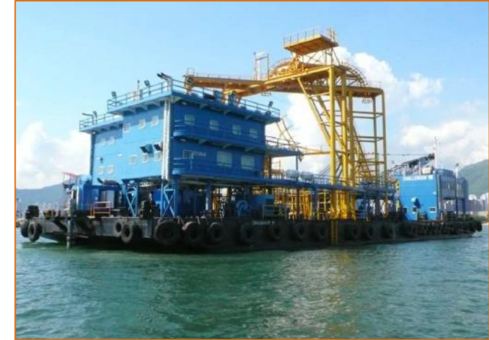
Typical Cable Installation Barge (Sledge Tool)
