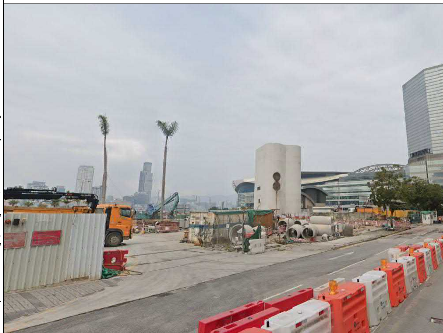
LR 5 – VEGETATION IN CONSTRUCTION WORKS SITE ON LUNG KING ROAD
