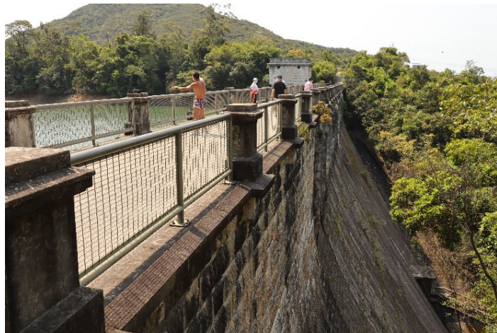
DM-02 – Aberdeen Upper Reservoir, Dam
