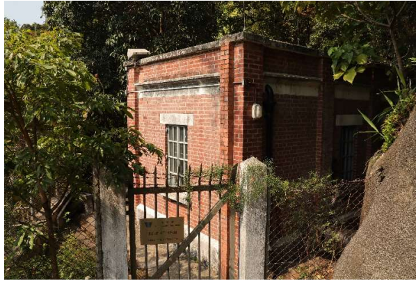
GB-01 – Aberdeen Reservoir, Lower Reservoir, Pump House
