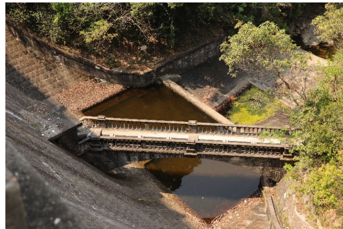
DM-04 - Aberdeen Upper Reservoir, Bridge
