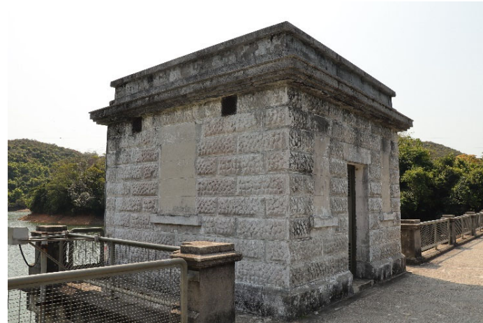
DM-03 - Aberdeen Upper Reservoir, Valve House
