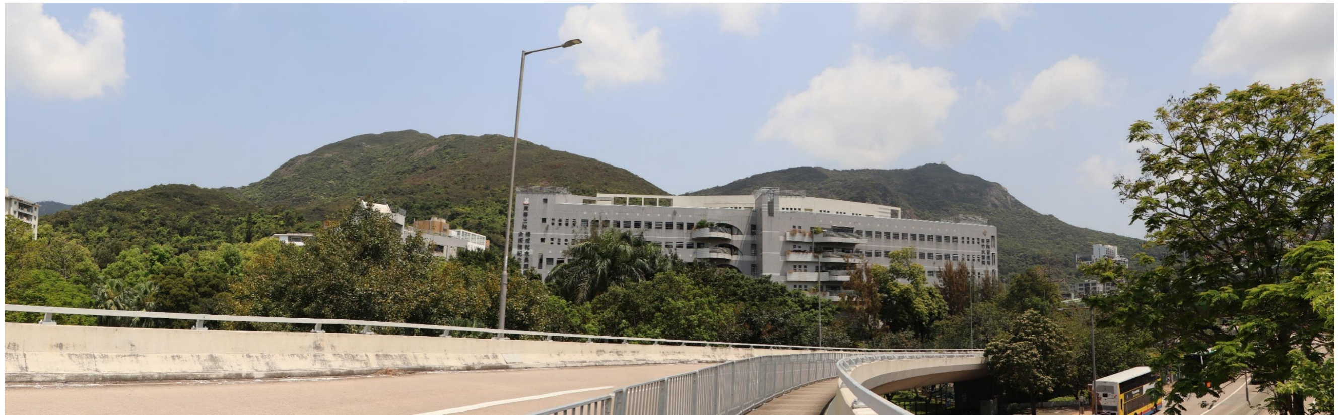
Day 1 after completion Viewpoint of PV 6 – View to Pylons from Wong Chuk Hang
