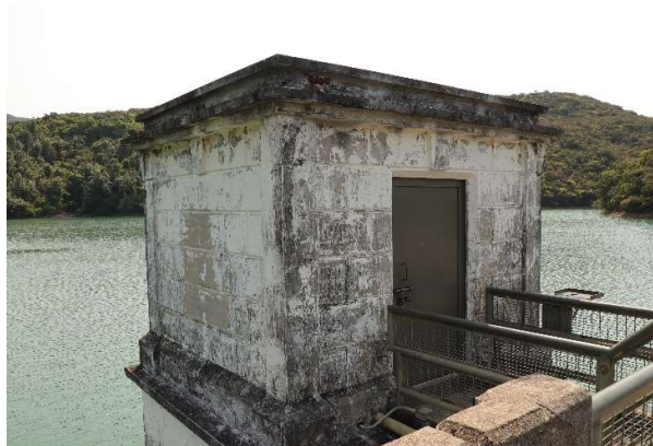
GB-02 - Aberdeen Reservoir, Lower Reservoir, Valve House
