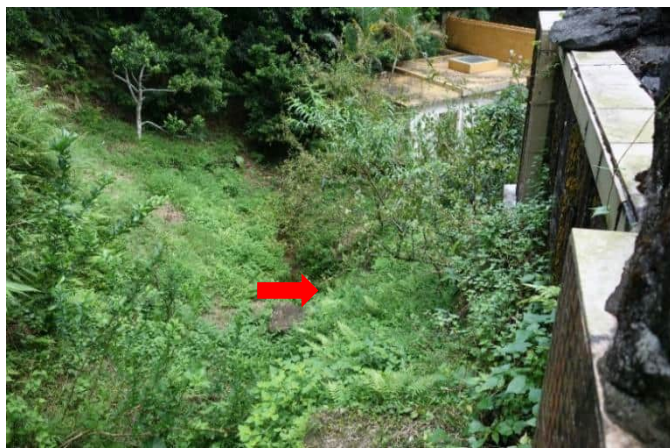
Plate 9 Natural Watercourse (S2) in the Surveyed Area
