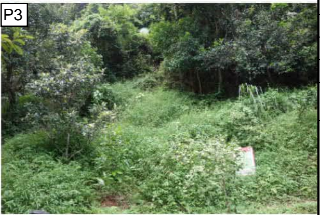
PLATE 3 - INDICATIVE LOCATION OF RIGID BARRIER RB01 相片3 - 泥石流RB01的指示性位置
