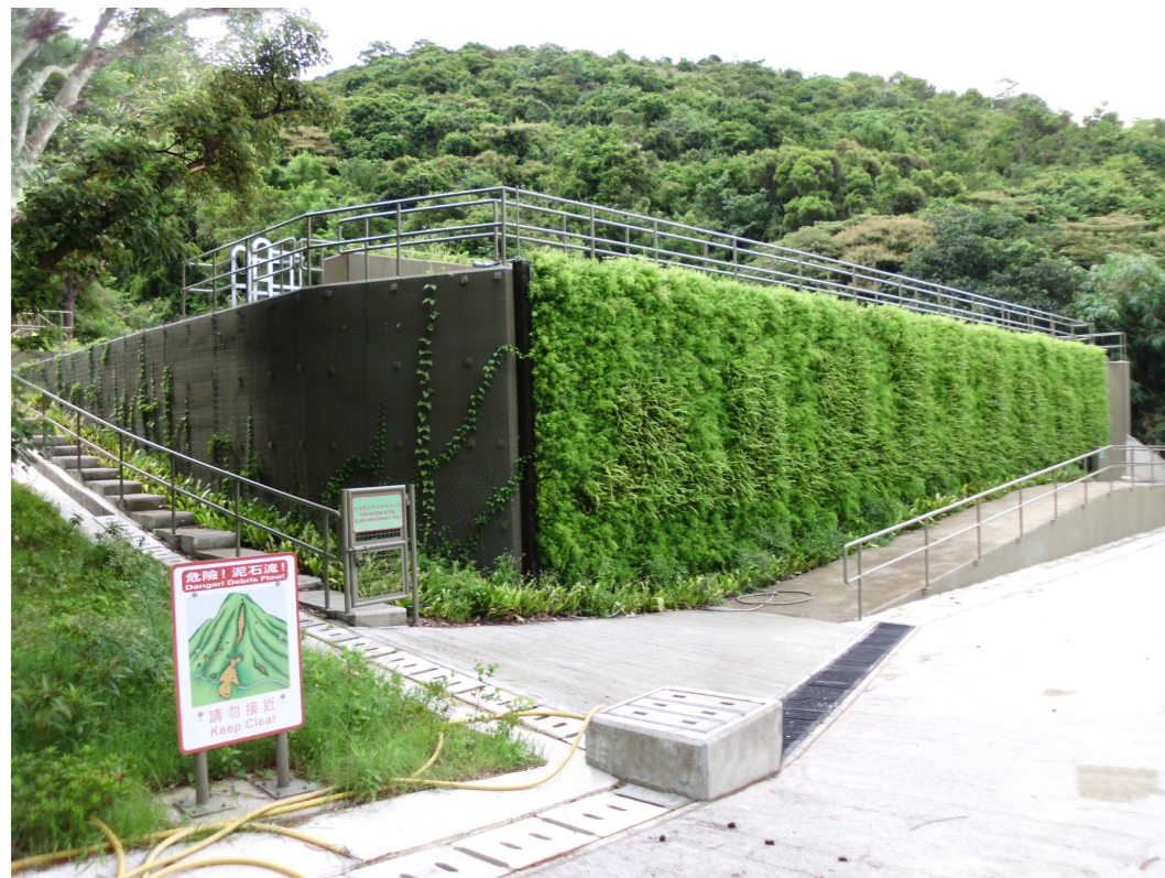
PREVIOUS EXAMPLES OF RIGID BARRIER FOR NATURAL TERRAIN HAZARDS MITIGATION WORKS 用於防治山泥傾瀉工程的泥石壩例子
