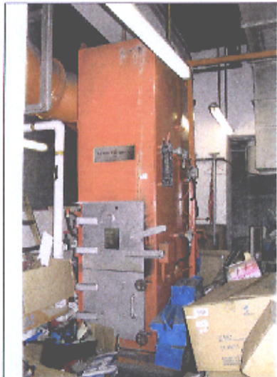
Incinerator to be demolished
