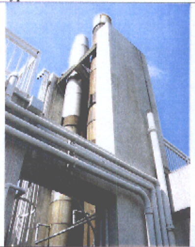
The top section of incinerator flue above roof level
