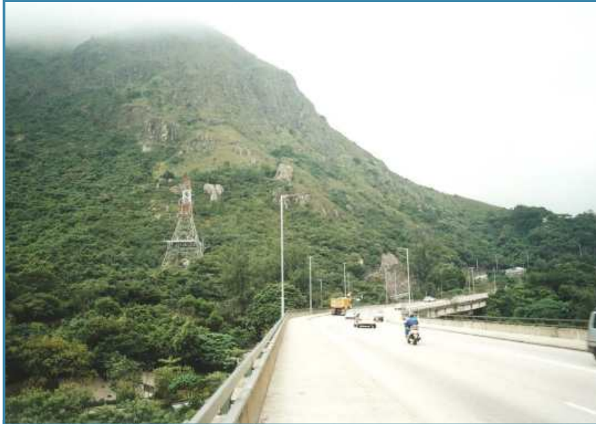
Plate 8 View from Flyover of New Clear Water Bay Road towards Tower 7.
