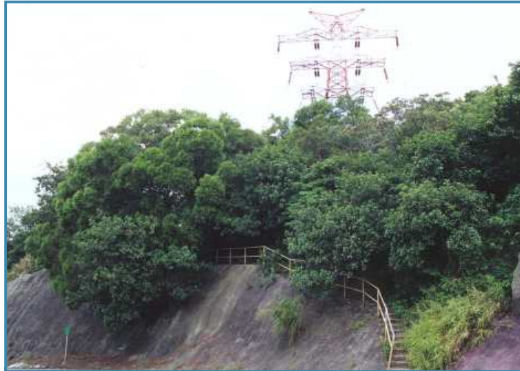
Plate 1 The Site viewed from Clear Water Bay Road. The cable alignment emerges from Ma On Shan Country Park between the base of the steps and the large boulder. (right of the picture)
