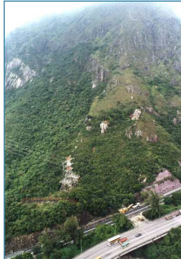
Plate 10 View from Roof of Shun Lee Discipline Services Quarter towards Tower 7.
