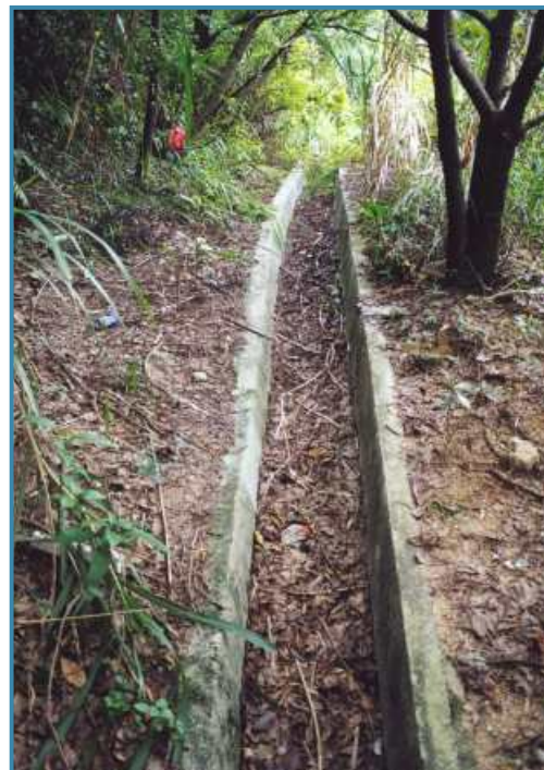
Plate 4 Sparse undergrowth on either side of the drainage channel.
