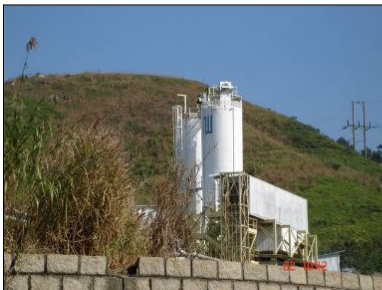
Photograph 4-7 K-Wah Concrete Batching Plant – Apparently Abandoned
