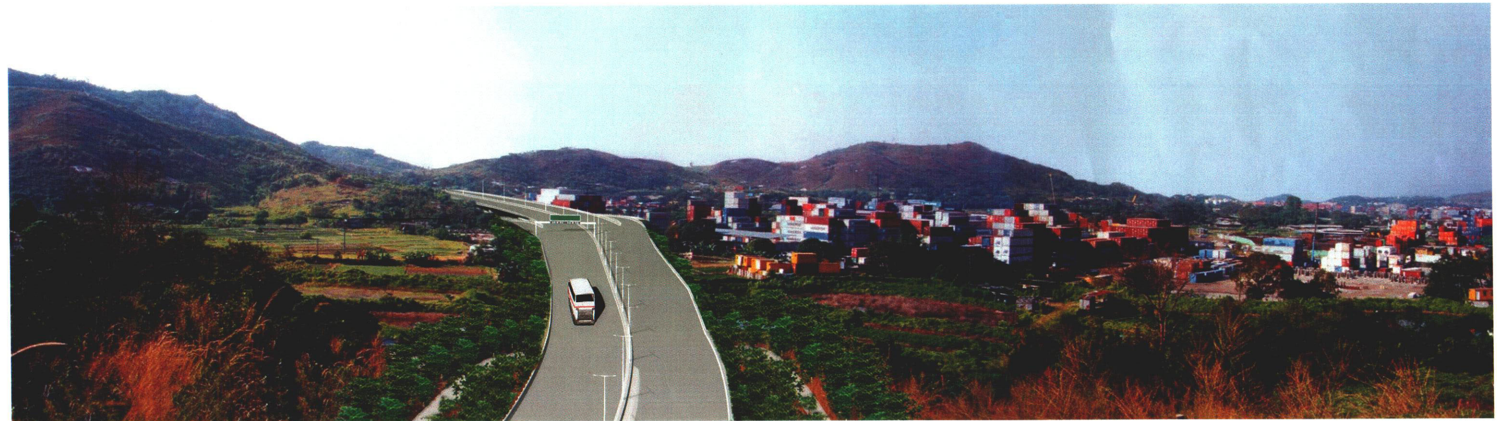
Photo View No. 5.4 Viewed from Hill East of Ha Tsuen - Year 10 With Mitigation
