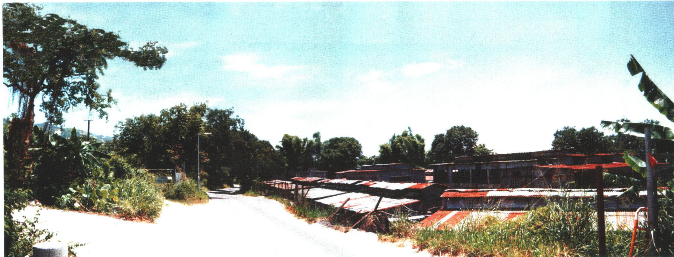
Photo View No. 8.1 Viewed from Deep Bay Road Looking West - Existing Condition
