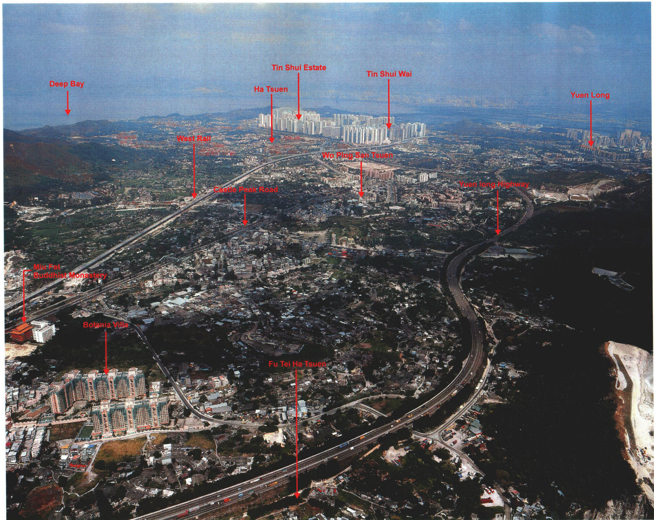
Aerial Photo View to Deep Bay Link- Existing Condition
