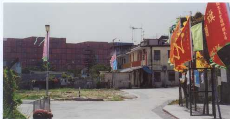
Viewpoint No. 11: Typical view towards San Wai STW from Tsueng Kong Wai. The STW is completely concealed behind the containers.
