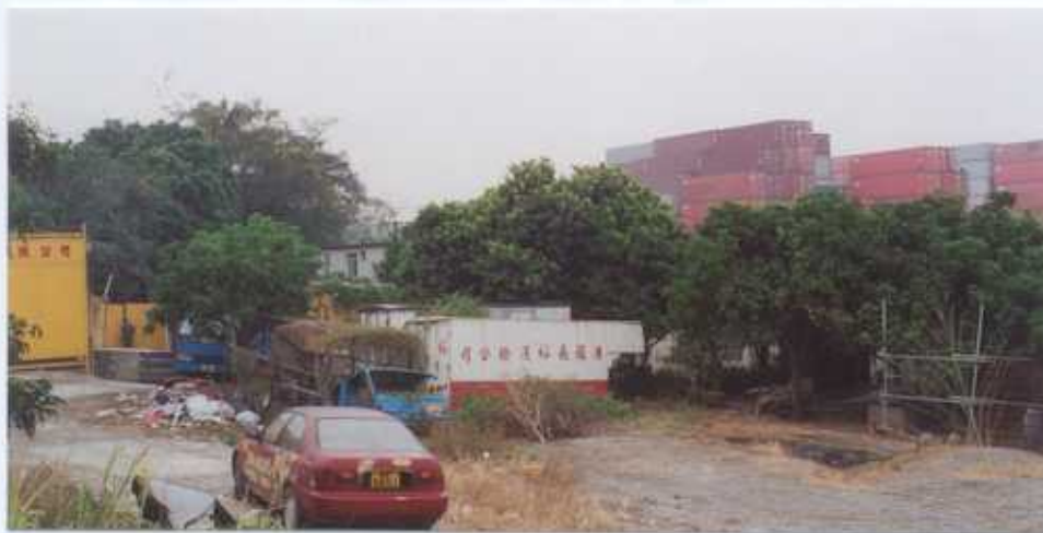
Viewpoint No. 9 Typical view towards San Wai STW from San Sang Tsuen. The STW is totally concealed behind the containers
