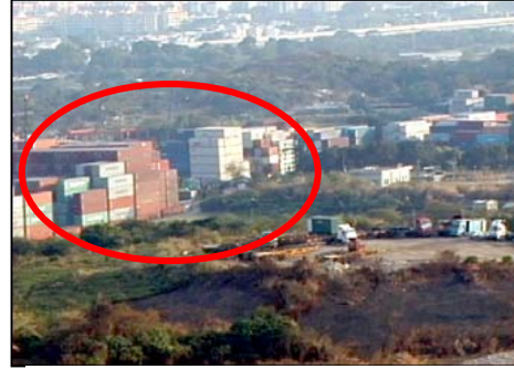
2. Container yard north-east of San Wai STW
