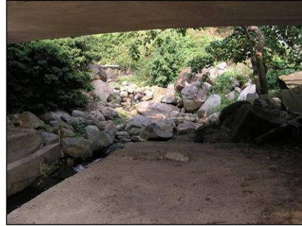
Underneath bridge crossing
