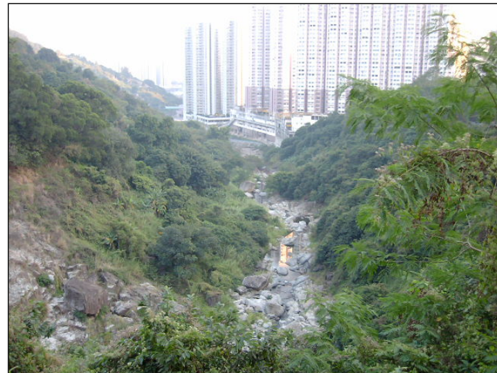
Most downstream of I-3
