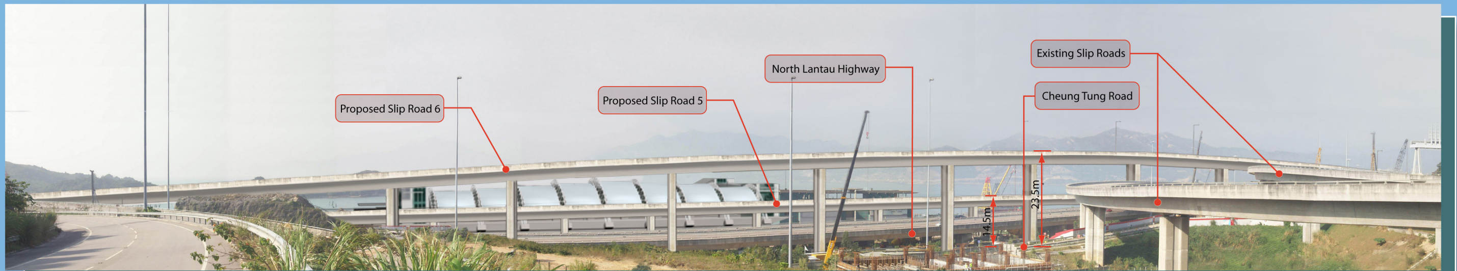
View North from Existing Link Road 1
