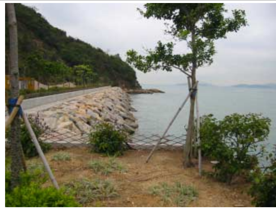
Granite Boulder Seawall (& Ornamental Planted area)
