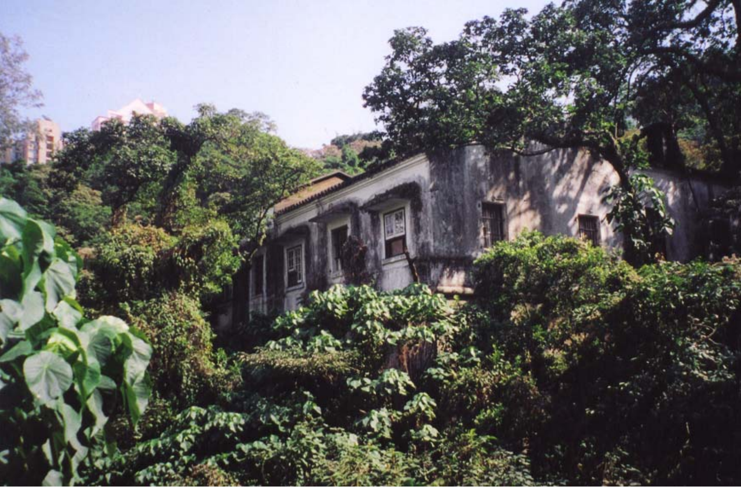
Figure 9.6 Partial Front and Side View of Laboratory Block of the Former Explosives magazine
