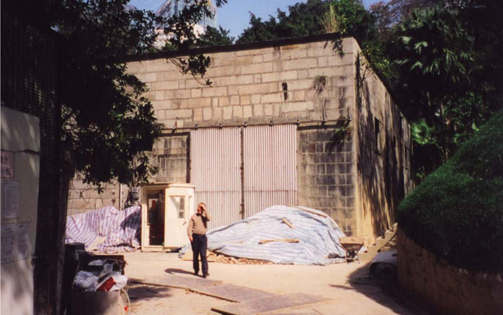
Figure 9.8 View of Magazine A, taken from the Entrance Gate
