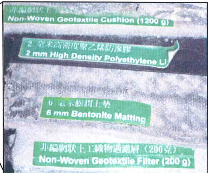
Cross-section of lining and leachate collection system
