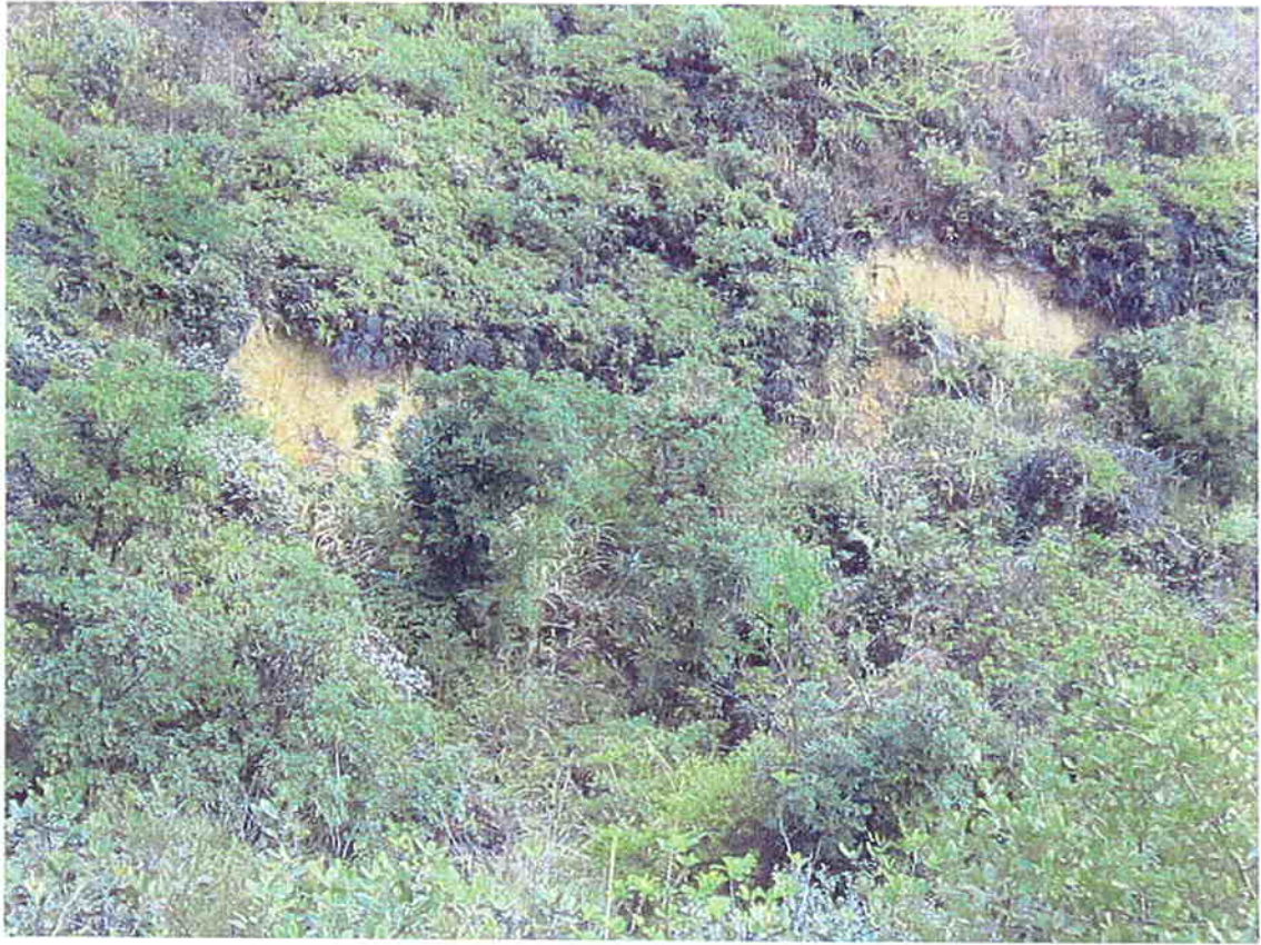
Plate 3: View of the Ngong Tong Study Area showing recent debris slide
