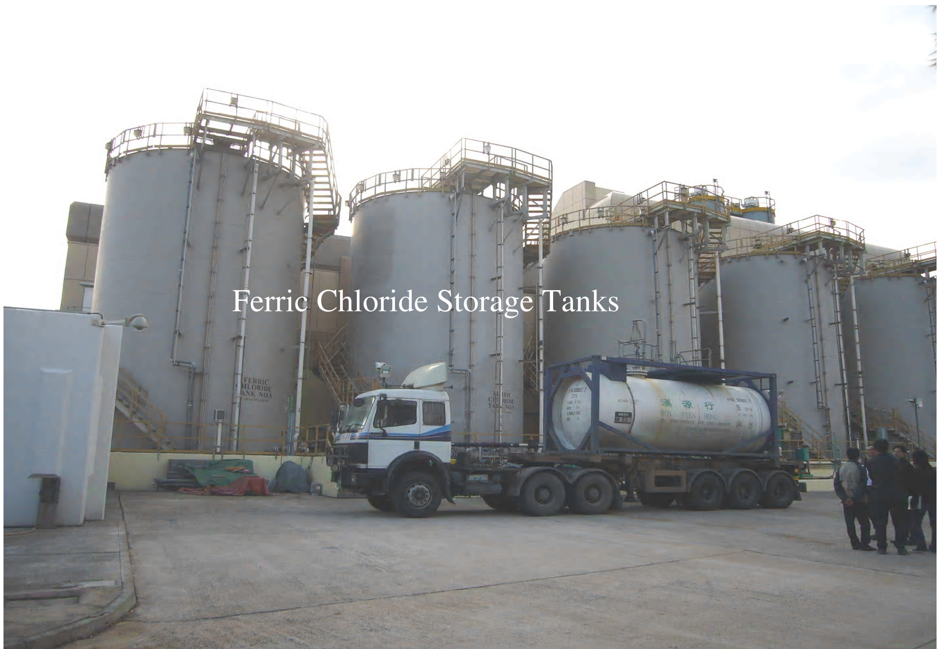
Ferric Chloride Storage Tanks
