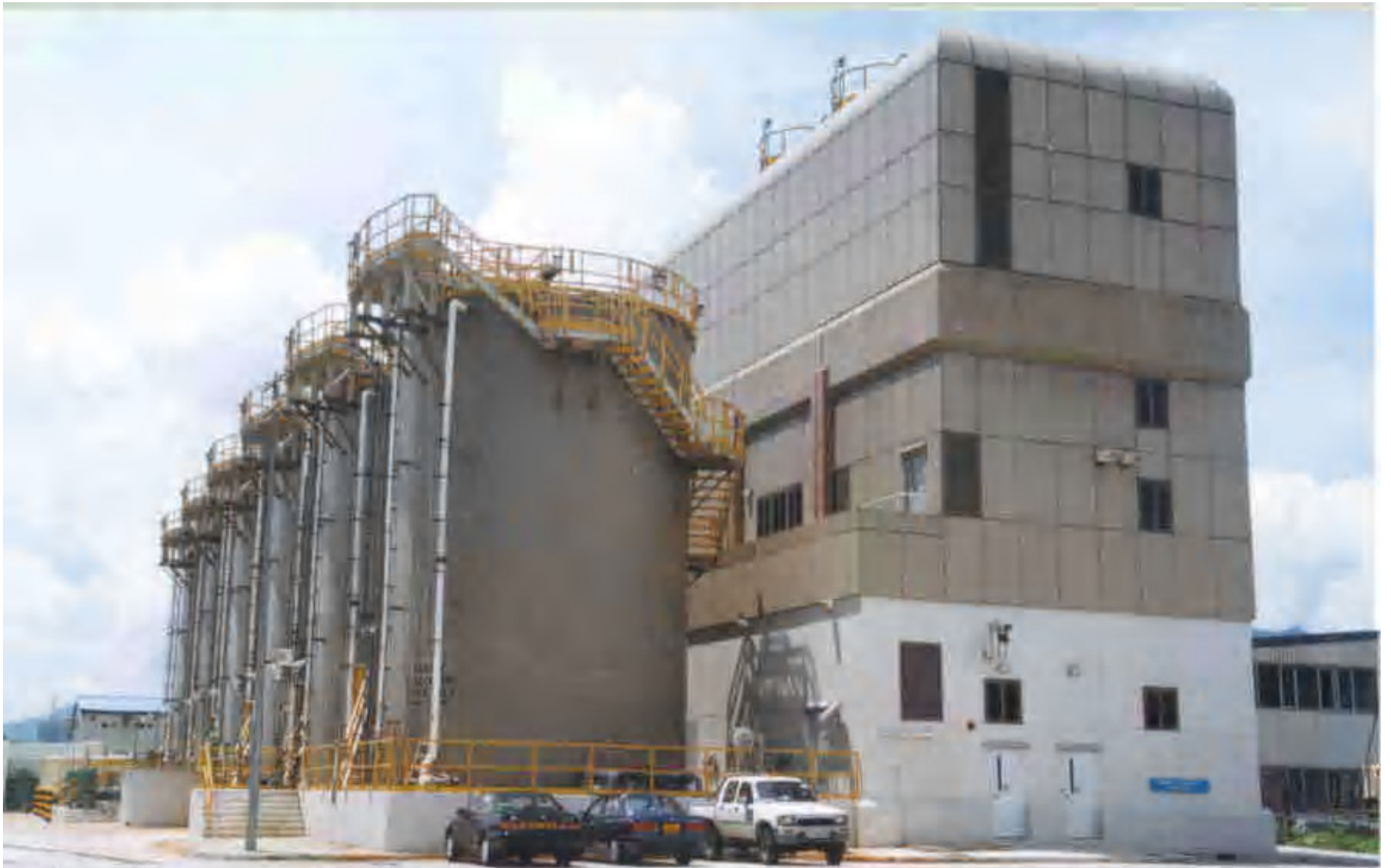
Ferric Chloride Storage Tanks
