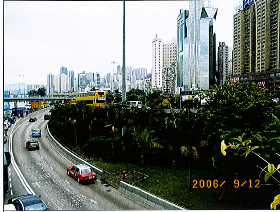
PHOTO A15 - LR9A TUNNEL APPROACH REST GARDEN
