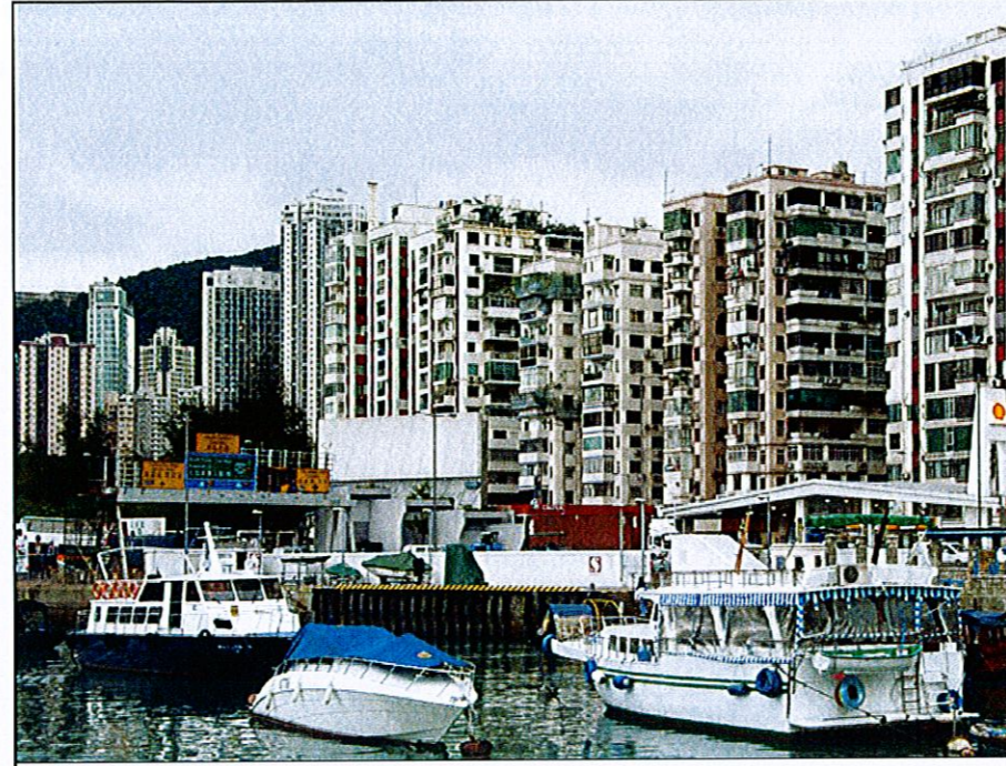
PHOTO A20 - LR13 WATERFRONT AREA ALONG CAUSEWAY BAY TYPHOON SHELTER
