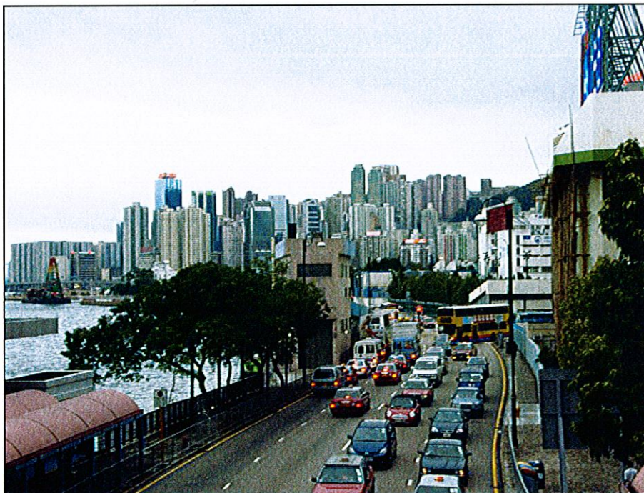
PHOTO A28 - LR20 STREET TREES ALONG CONVENTION AVENUE AND HUNG HING ROAD
