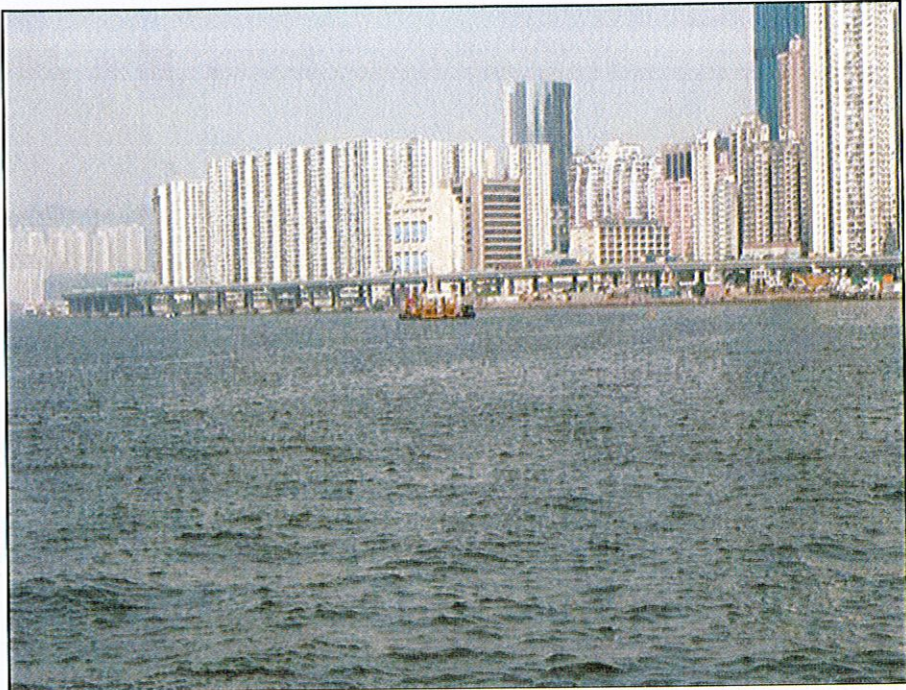
PHOTO C20 - T3 ISLAND EASTERN CORRIDOR
