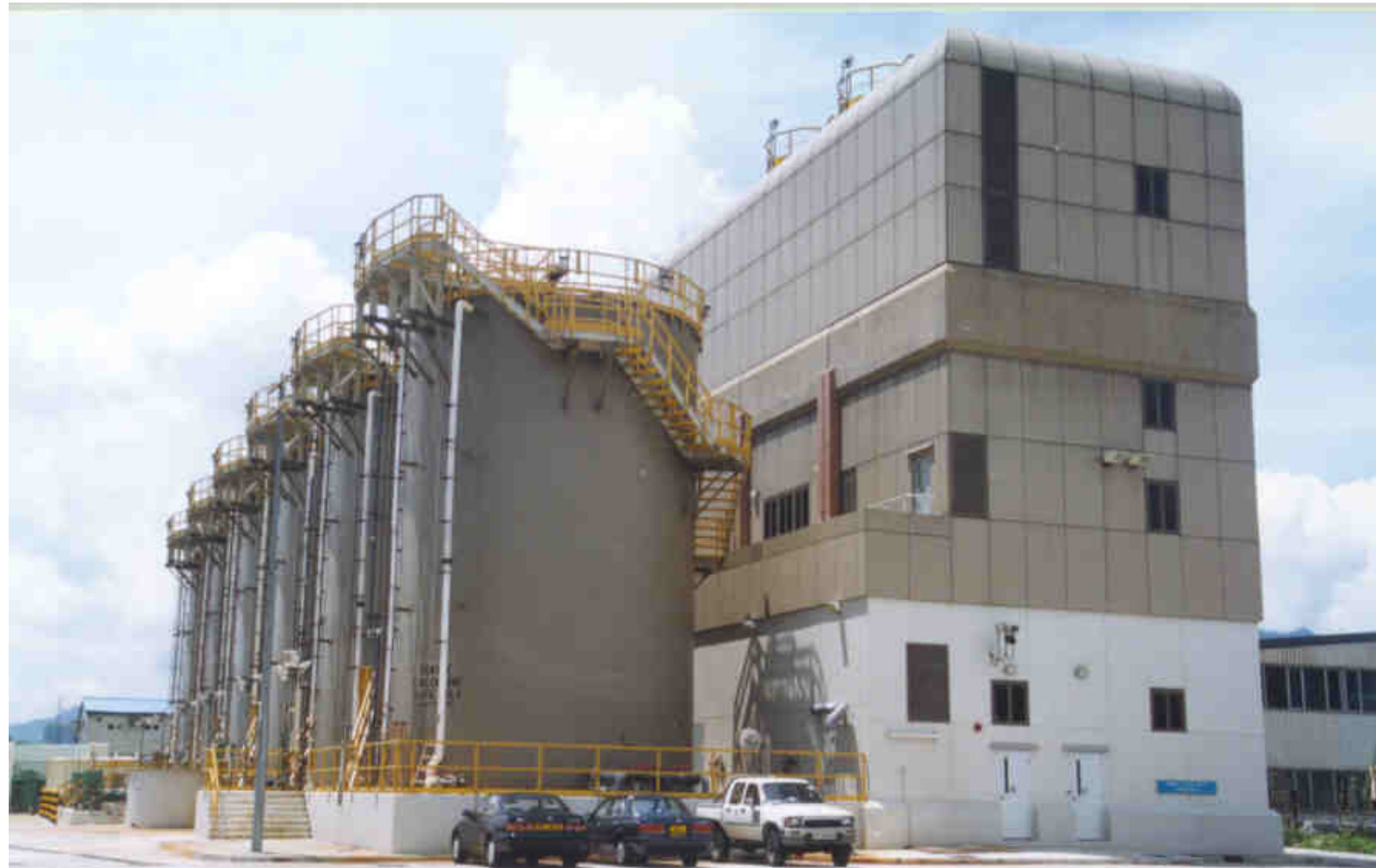
Ferric Chloride Storage Tanks Chemical Dosing Building
