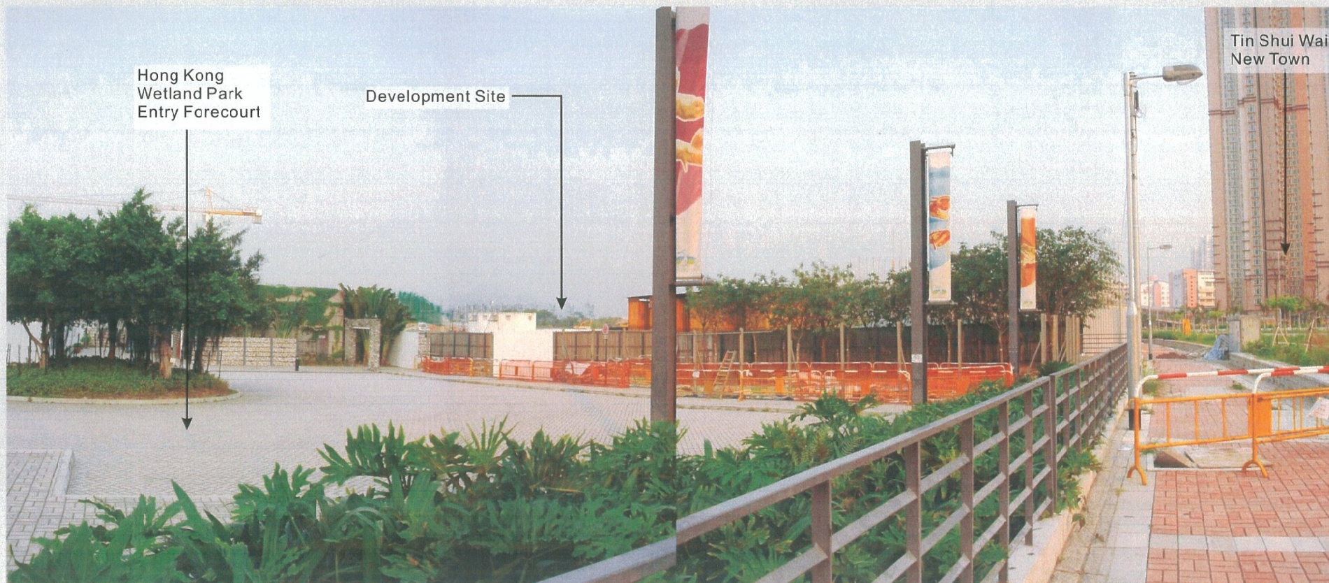
Year 1 of Operation Phase without landscape mitigation measures View southeast from the Hong Kong Wetland Park Entry Forecourt (VSR13)
