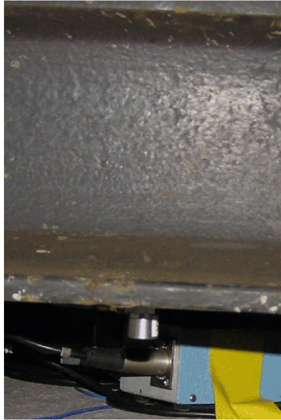
PHOTO 2 WILCOXON ACCELEROMETRE INSTALLED UNDER THE HIGH AND LOW RAIL
