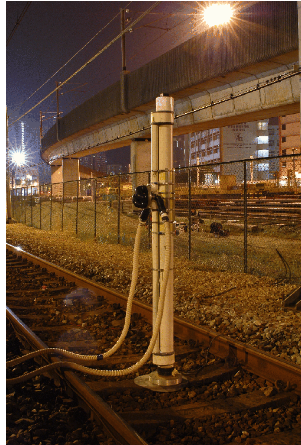
PHOTO 1 WHAMMY IMPACTING WITH A HAMMER PLATFORM INSTALLED ON TOP OF A CONCRETE SLEEPER TO TRANSMIT THE IMPACT FORCE TO THE BALLAST TRACK
