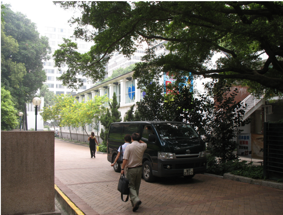
View of the North facing elevation of Block S4 taken from Kowloon Park
