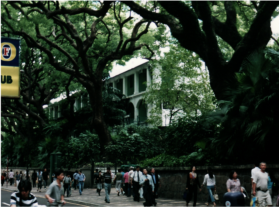
View of Block S58 (Southern elevation) from Haiphong Road
