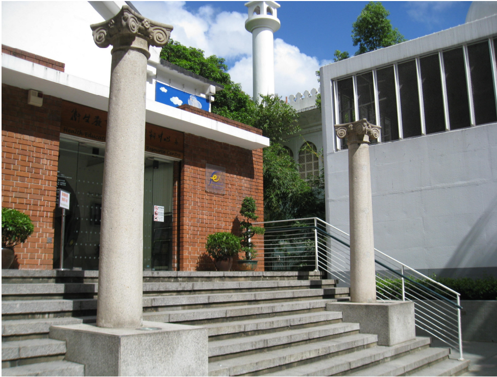
Two granite columns removed from Eu Yan Sang Medicine company on the steps leading up to the current entrance of the building
