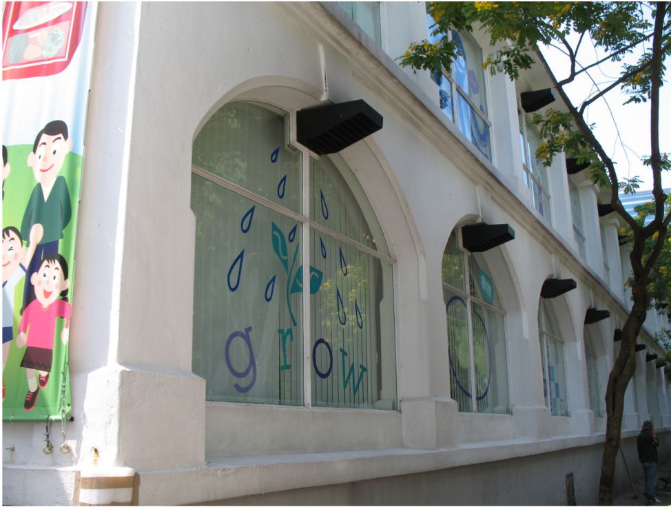
View of the Northeastern corner of Block S4 showing the modern windows
