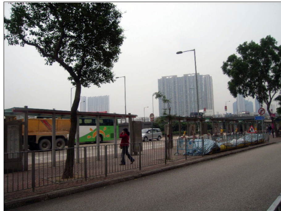
PHOTO D07 - R3 FROM LOW TO MEDIUM-RISE RESIDENTIAL DEVELOPMENT IN KOWLOON CITY
