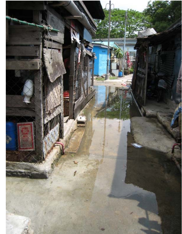
Plate 9 Localised flooding within Hang Hau Tsuen during high tide.
