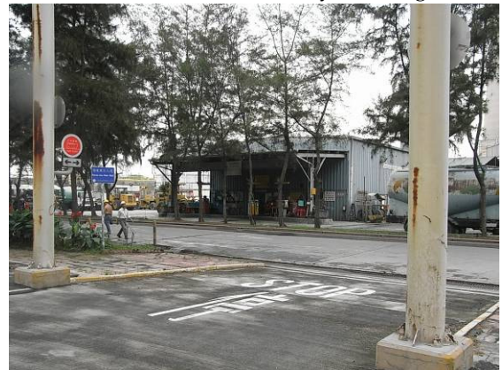
Photo 6 – Fuel USTs and dispensing station
