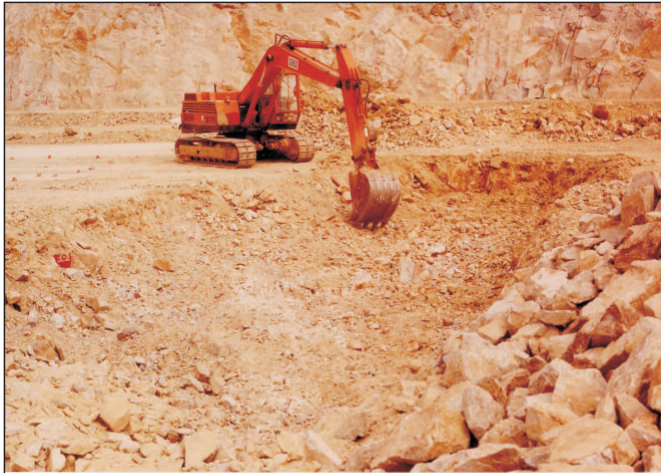
FINISH GRINDING AREA – FINISH MILL FOUNDATION EXCAVATION DECEMBER 11, 1980.
