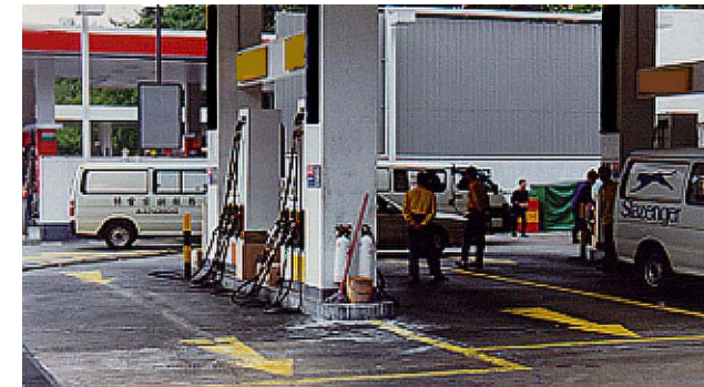
Figure 1.2 – Petrol Filling Stations
