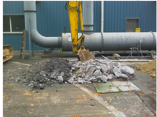
Photo 4 – Excavation at S3/S4
