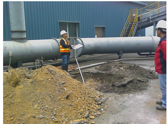
Photo 6 – Identification of soil profile by contractor
