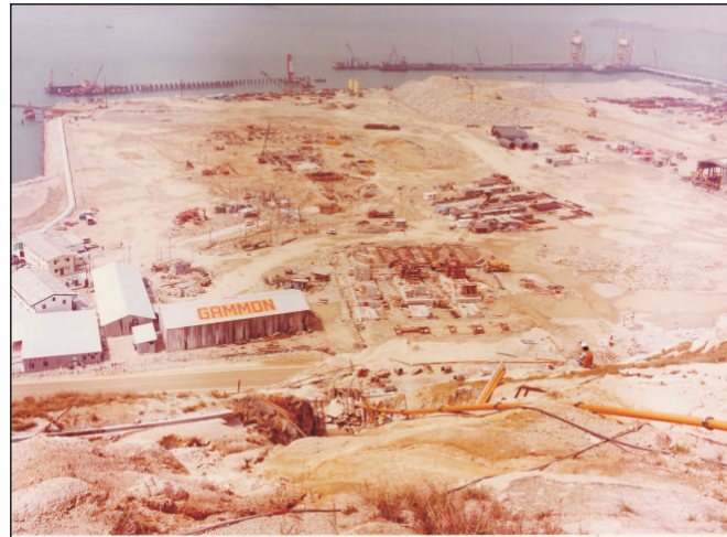
GENERAL VIEW OF SITE LOOKING SOUTH, MARCH 21, 1981.
