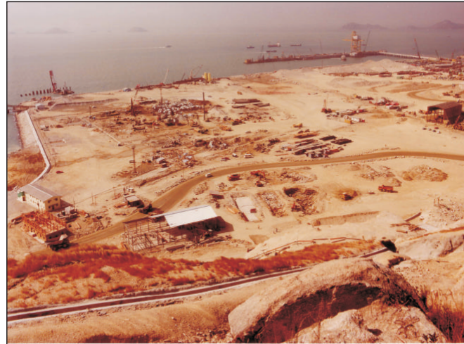
GENERAL VIEW OF SITE LOOKING SOUTH. JANUARY 22, 1981.
