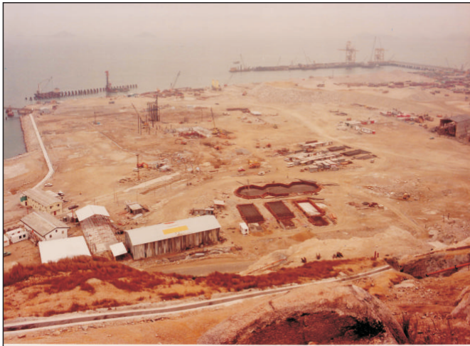
CASTLE PEAK CEMENT PROJECT SITE. FEBRUARY 27, 1981
