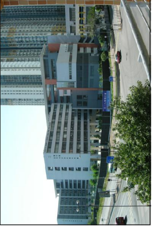
GIC 9.1 Schools along Hing Wah Street West: SKH St. Mary's Church Mok Hing Yiu College, SKH St. Andrew's Primary School, Tsung Tsin Christian Academy and Tack Ching Girls' Secondary School
