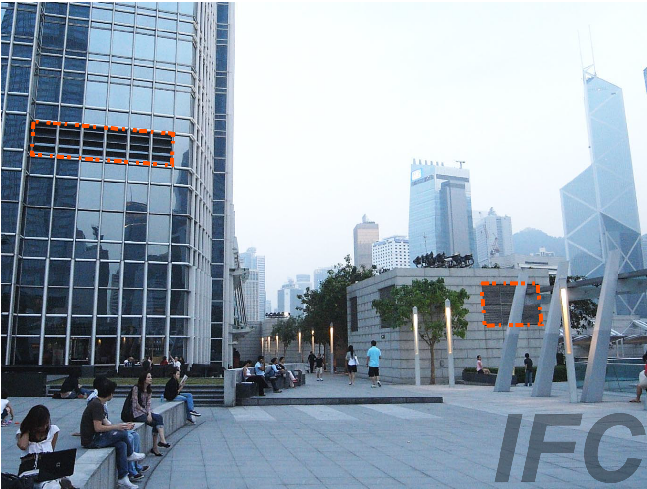
Louvres for HK Station - Design interface to be matched with façade wall and overall colour scheme of the place; located above pedestrian level to avoid adverse impact for recreational user.
