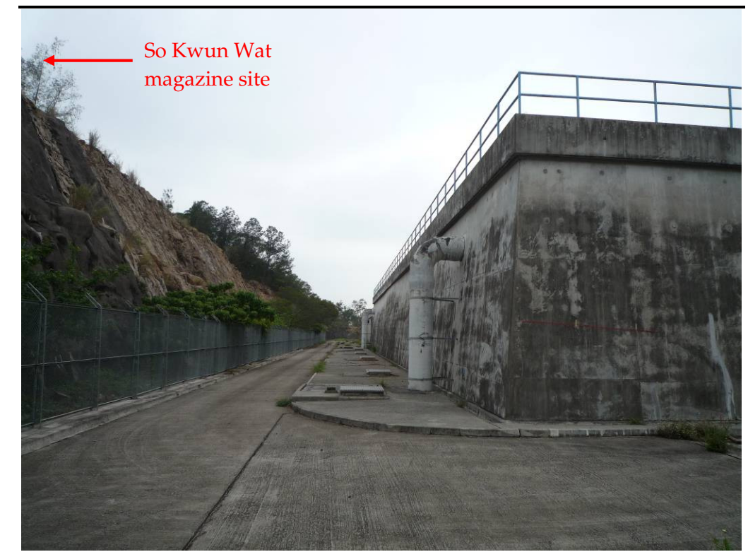
Figure 7.2 Siu Lam Fresh Water Storage Tanks
