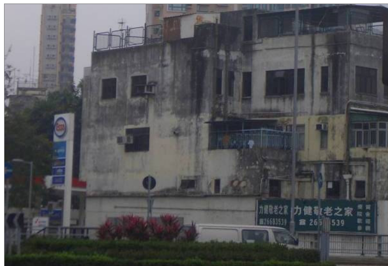
▪ Photo 62 N17 (Shing Fat Building)
