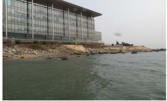
Natural Bedrock at D4
