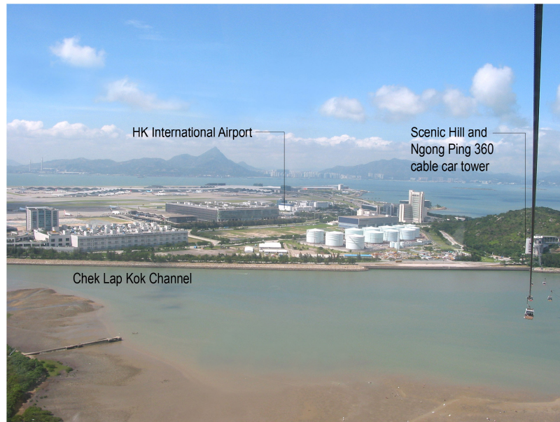
Existing Baseline Condition
