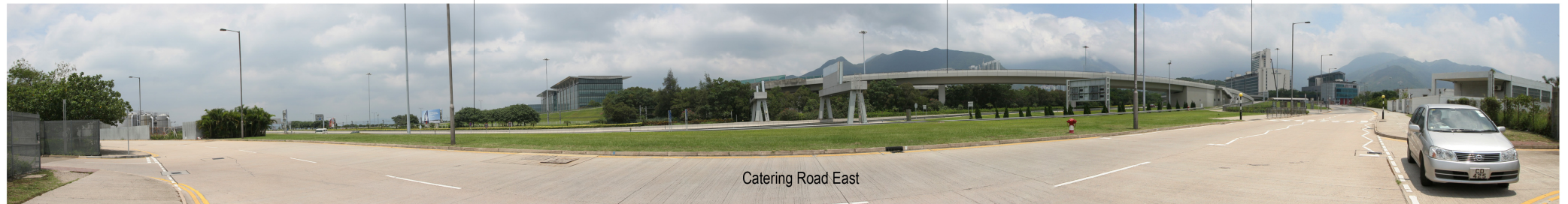
Existing Baseline Condition
