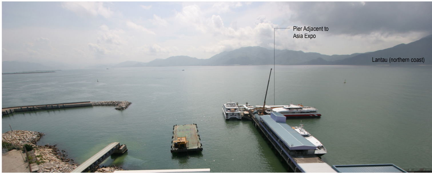
Existing Baseline Condition
